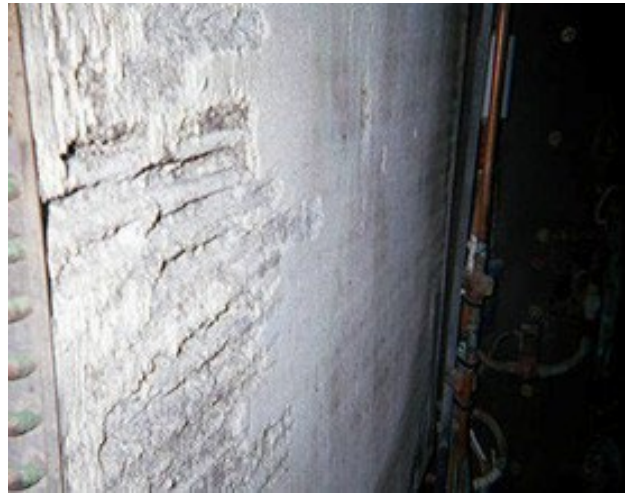
Corroded Dehumidifier
